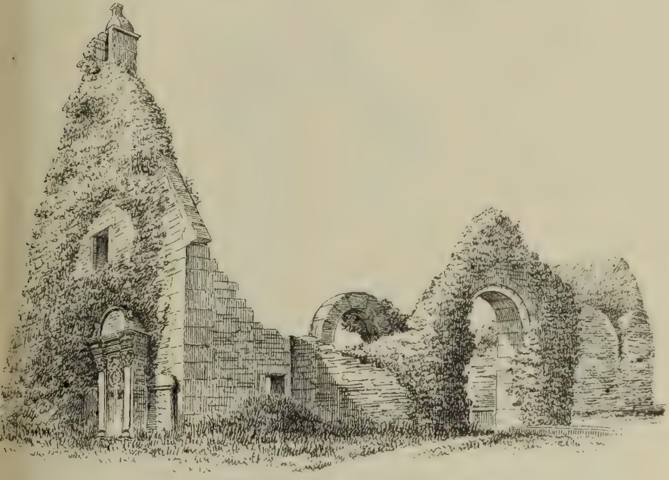
FIG. 1375.—Carnock Church. View from South-West.
